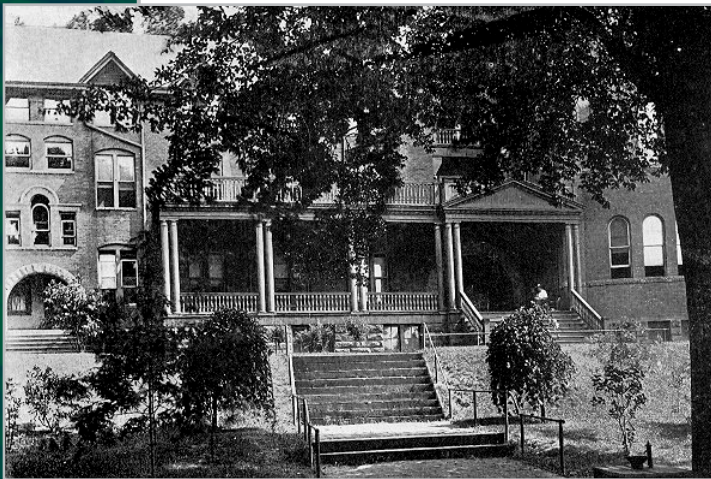
College Hall's Veranda, built in 1848, is now Old Main's north side. The double stairs in the foreground still exist.
